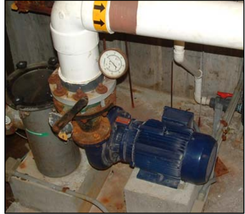
Fig 7. Recirculation pump
