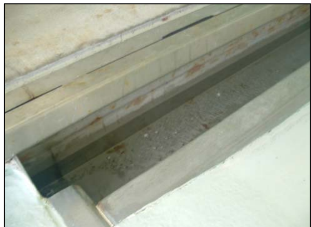
Fig 3. Sand/media in gutter trough
