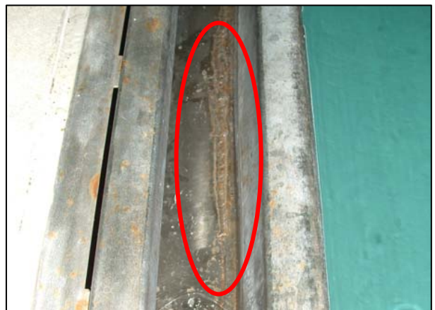
Fig 4. Leaking seam
