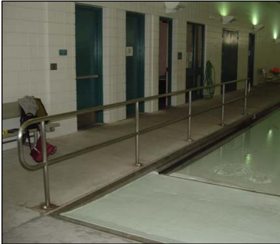
Fig 11. Loose handrail
